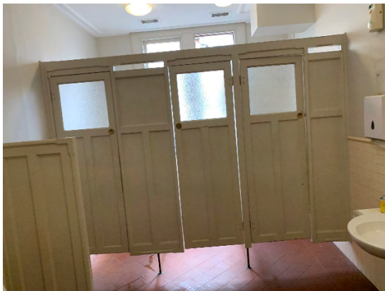
Figure 11 – Early bathroom partitions on second floor of 94 Oxford Street.
